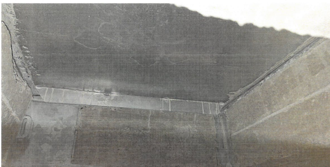
Figure 2: Watertightness test – no water penetration
