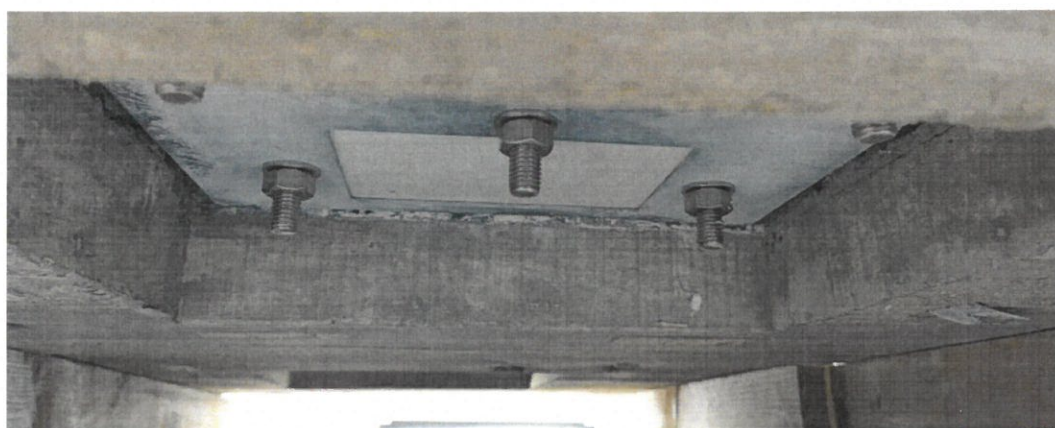
Figure 2: Watertightness test – no water penetration
